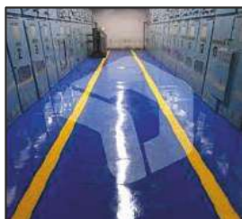
EPOXY FLOOR COATING
