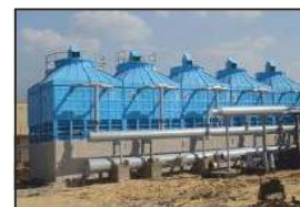
COOLING TOWER & CONCRETE TANK COATING
