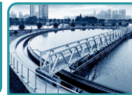
Waste Water Treatment
