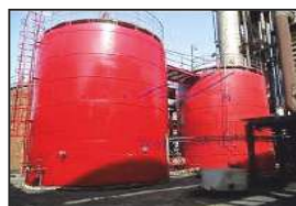
INTERNAL & EXTERNAL TANK COATING
